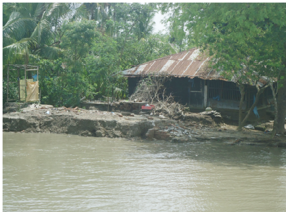
Loss of house due to riverbank erosion
