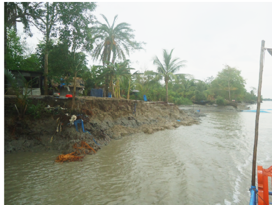
Loss of house due to riverbank erosion
