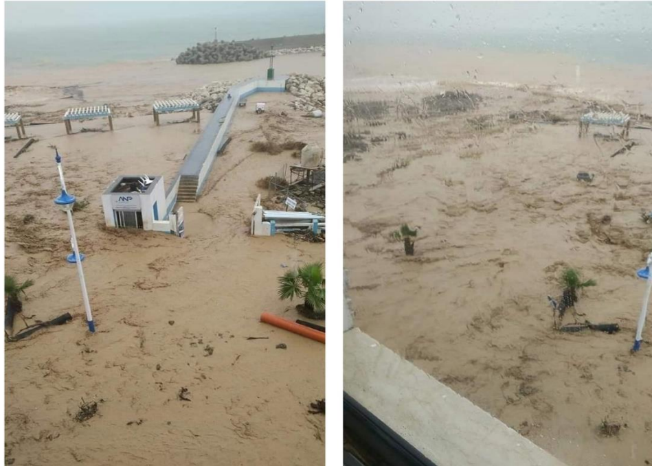
Figure 2: Images of flood impacts on Jebha Port
